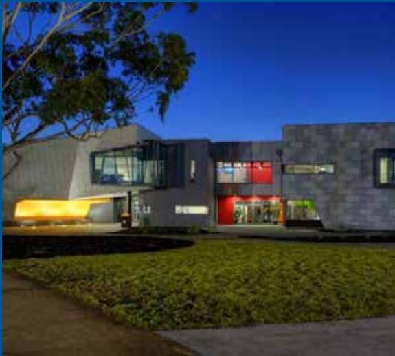
Above: Located in Boundary Road, just 10 minutes' drive from The Gordon's Geelong City Campus, our spacious East Geelong Campus is the trade training hub where all trade courses are delivered. The campus offers ample free parking and is home to quality training facilities including the new Renewable & Clean Energy Innovation Training Hub currently under development.
